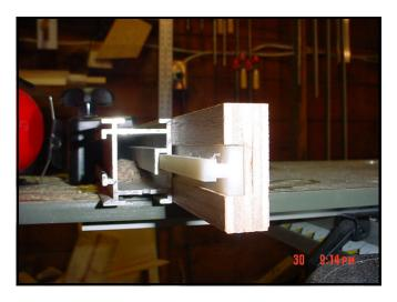
Attach the plastic to the plywood using #4-3/4'' flat head wood screws through the plywood into the plastic in pre-drilled counter sunk holes.
